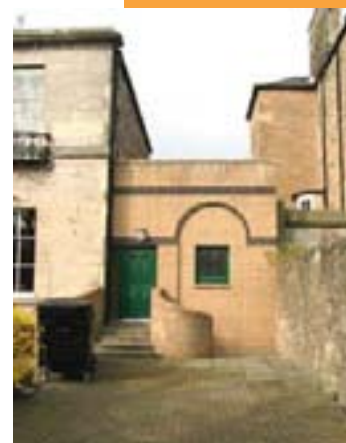
Ground floor extension
