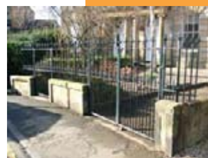
Railings at Blacket Place
